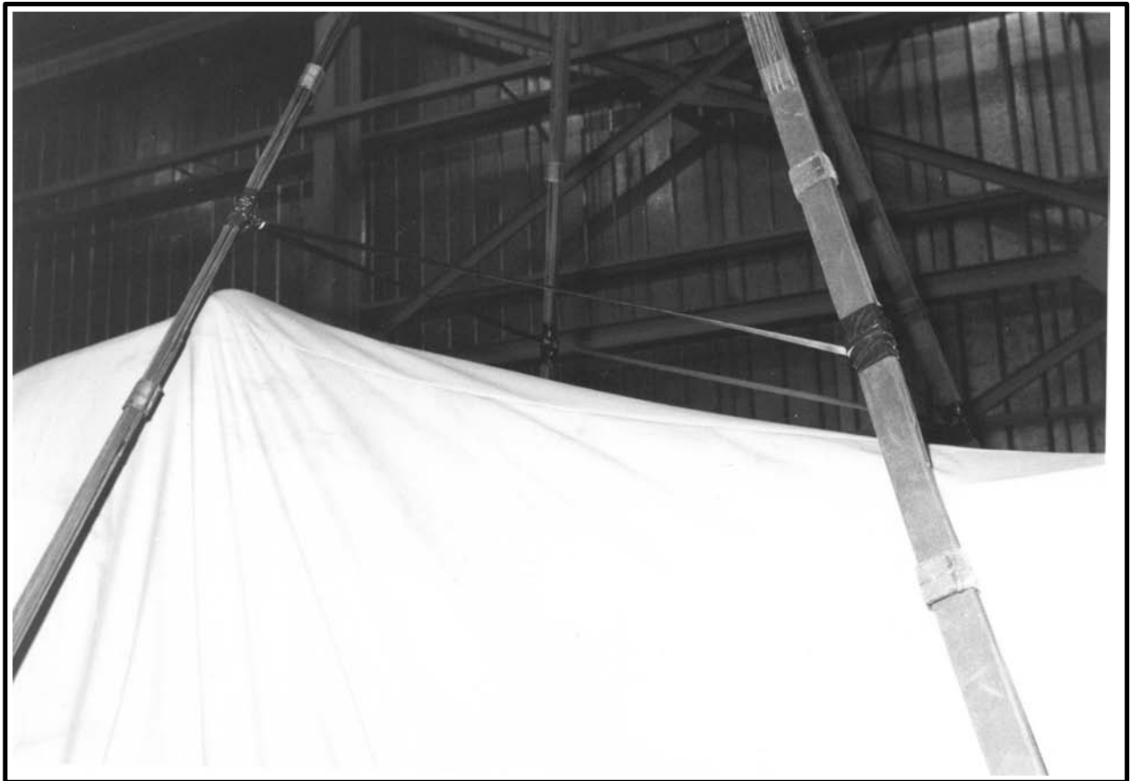
Figure 4-24 Deadman Ties Installed
