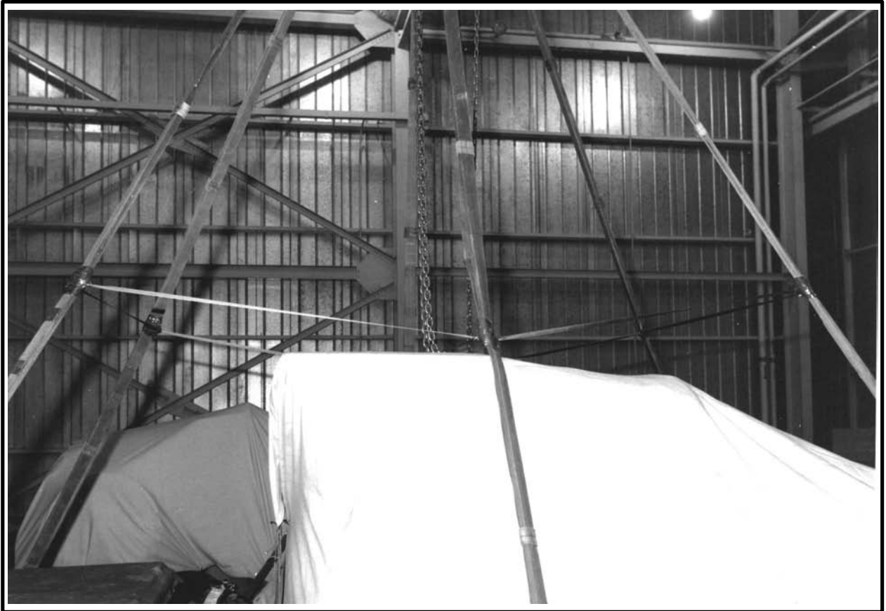
Figure 8-17 Deadman Ties Installed
