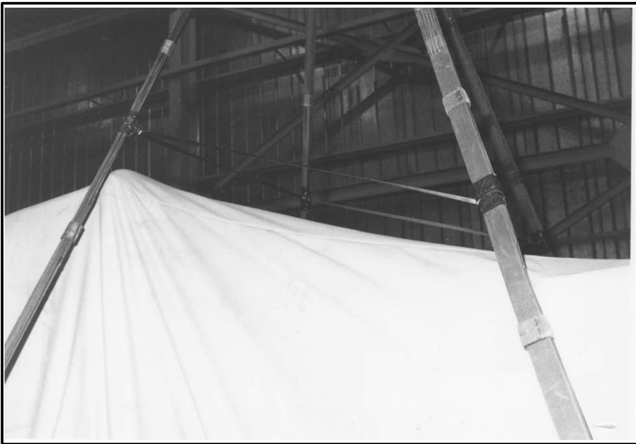
Figure 6-32 Deadman Ties Installed
