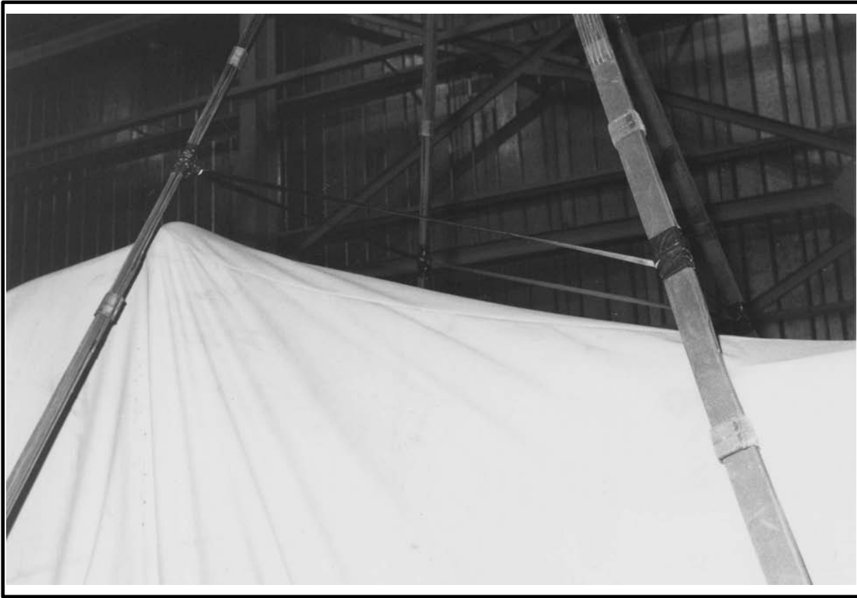
Figure 2-8 Deadman Ties Installed
